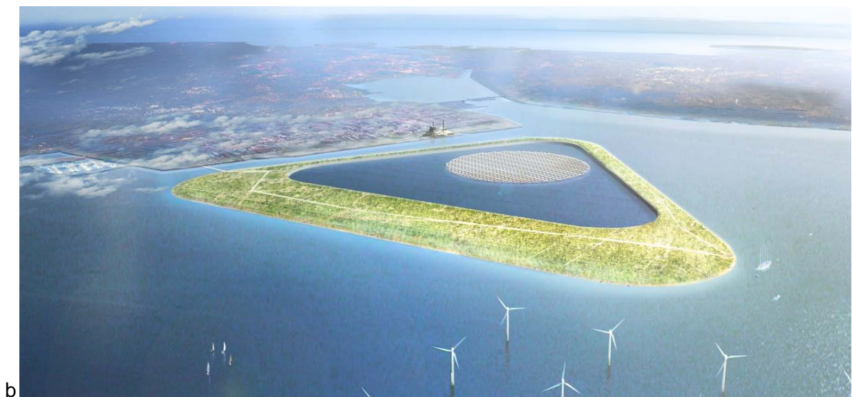
Figure 3.4.2. Artistic drawing of an Energy Island 24 . Water from the deep interior of the island is pumped out in periods of surplus electricity. The electricity can subsequently be regenerated when water is allowed to flow back via turbines. The concept may be expanded with wind turbines (on-shore foundations), solar cells (circle in the middle) as well as algae production.
