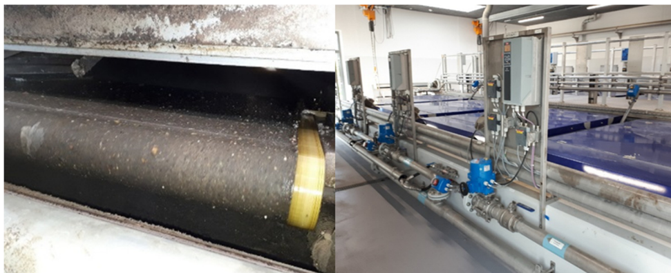
Figure D - 2: Photos of the Salsnes filter installation of Egaa WWTP
