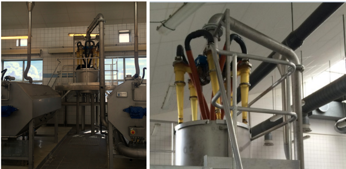
Figure 5: Hydrocyclone installation at Egaa WWTP
