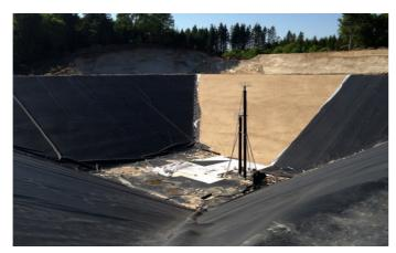
The storage in Dronninglund is situated in an abandoned gravel pit. This made the excavation easy compared to Marstal, where clay caused problems as excavation took place in a rainfull summer.
