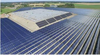
The storage is charged to  $85^{\circ}$  C during summer and discharged to  $10^{\circ}$  C during winter. The storage is used directly and as heat source for the compressor driven heat pump.
