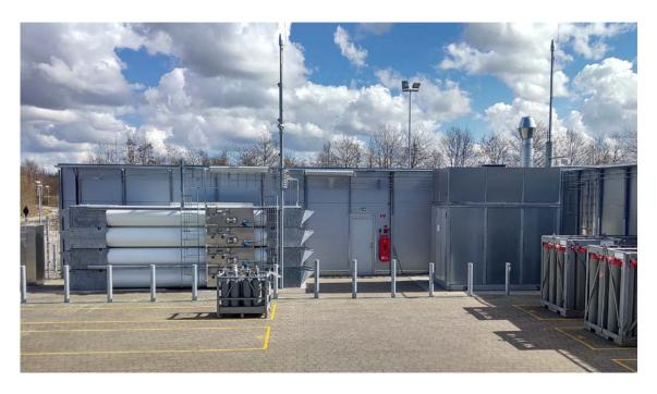
The HRS is connect to two dispensers placed outside of the test yard, in an area with public access. Picture below shows the two dispensers placed side-by side. The co-location allows for both LDVs and HDVs to be fueled at the same location.
